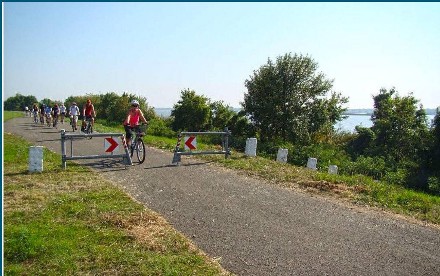
Lake Tisza dam
